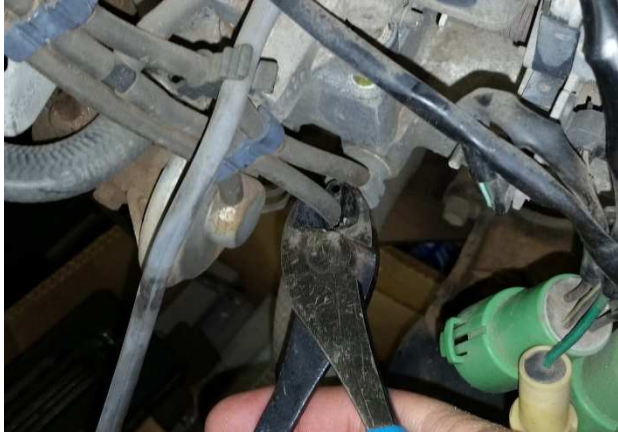
Cut vacuum lines from Thermo Switch
