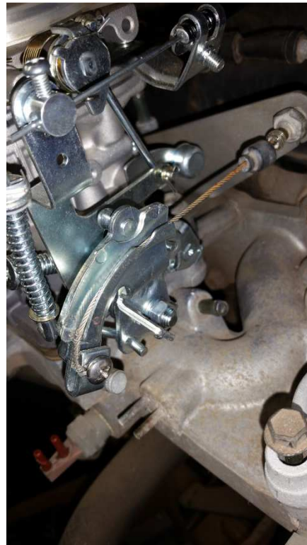
Allow cable to lay in groove
